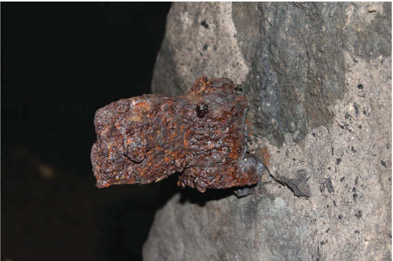
Plate 6: Former gated entrance, detail of rusted hinge in the east side, from the north-east
