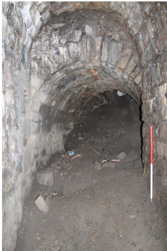
Plate 10: Entrance Passage, general view from the south
