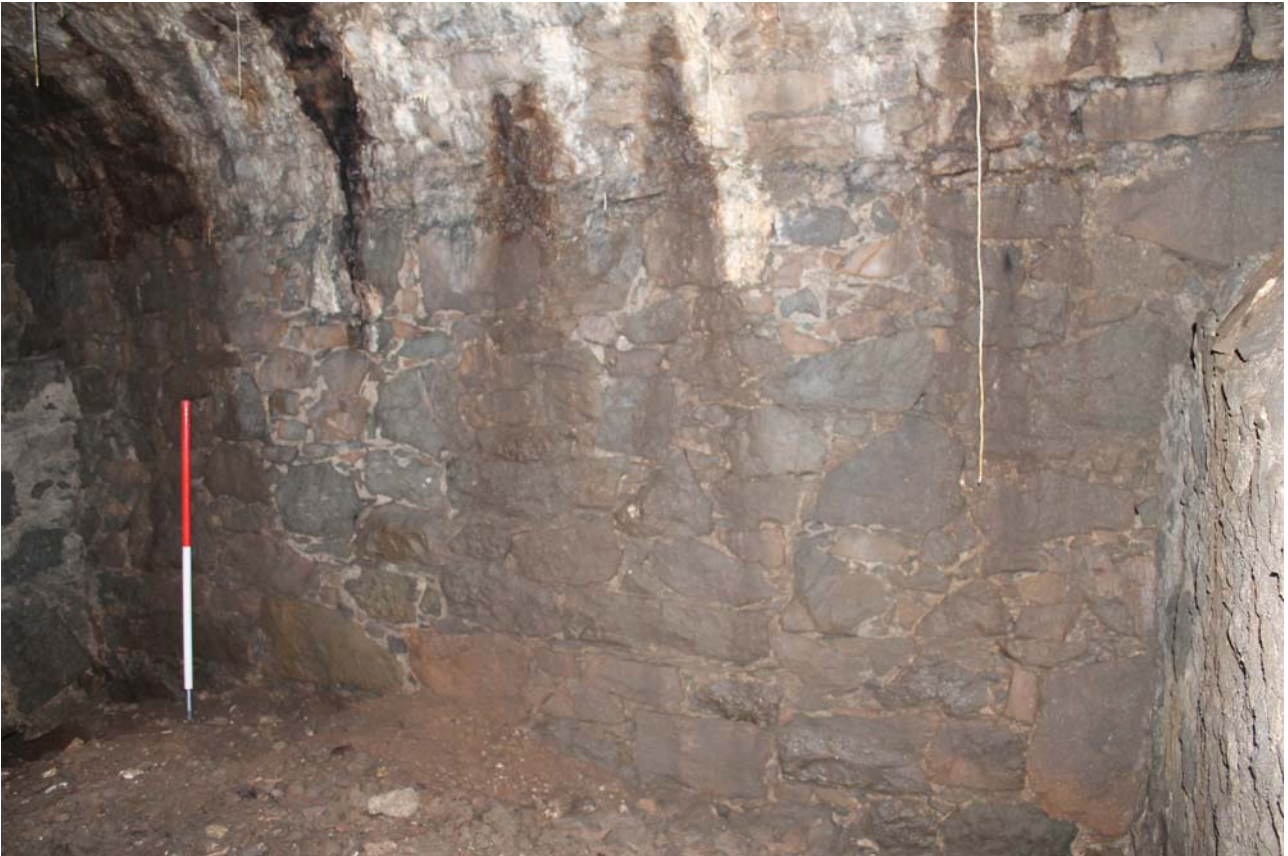
Plate 3: Main Chamber, general view of the south wall from the north-west
