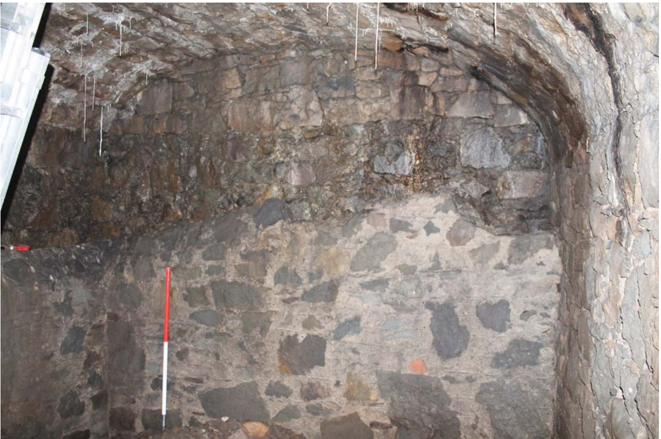
Plate 2: Main chamber, general view of the east wall from the west
